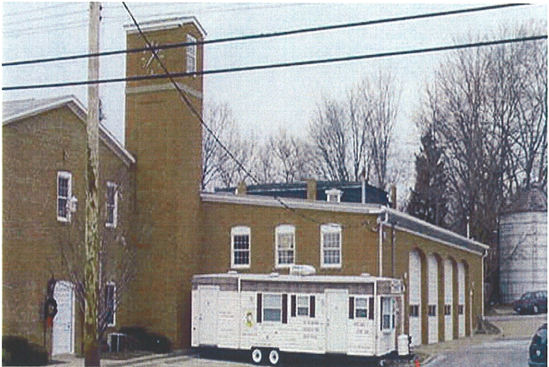
Photo #5: Oxford Fire Station, Rear View
