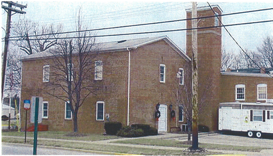
Photo #4: Oxford Fire Station, Side View
