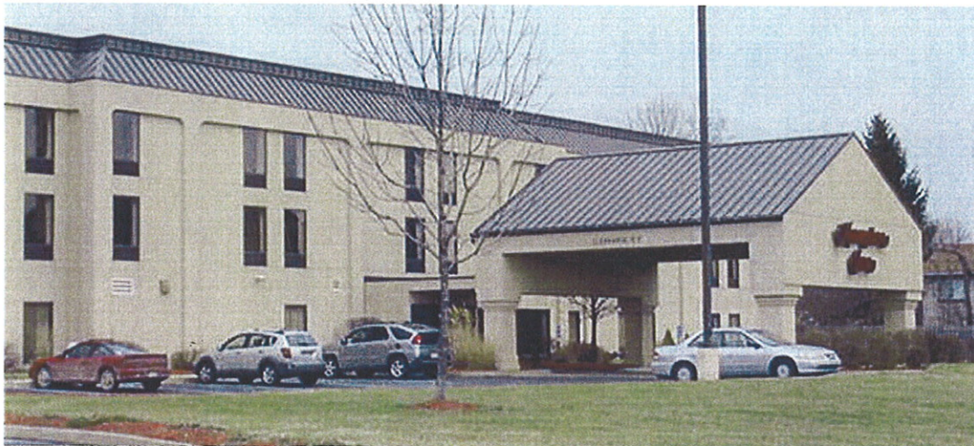
Photo #37: New Hotels are Being Constructed in the Area
