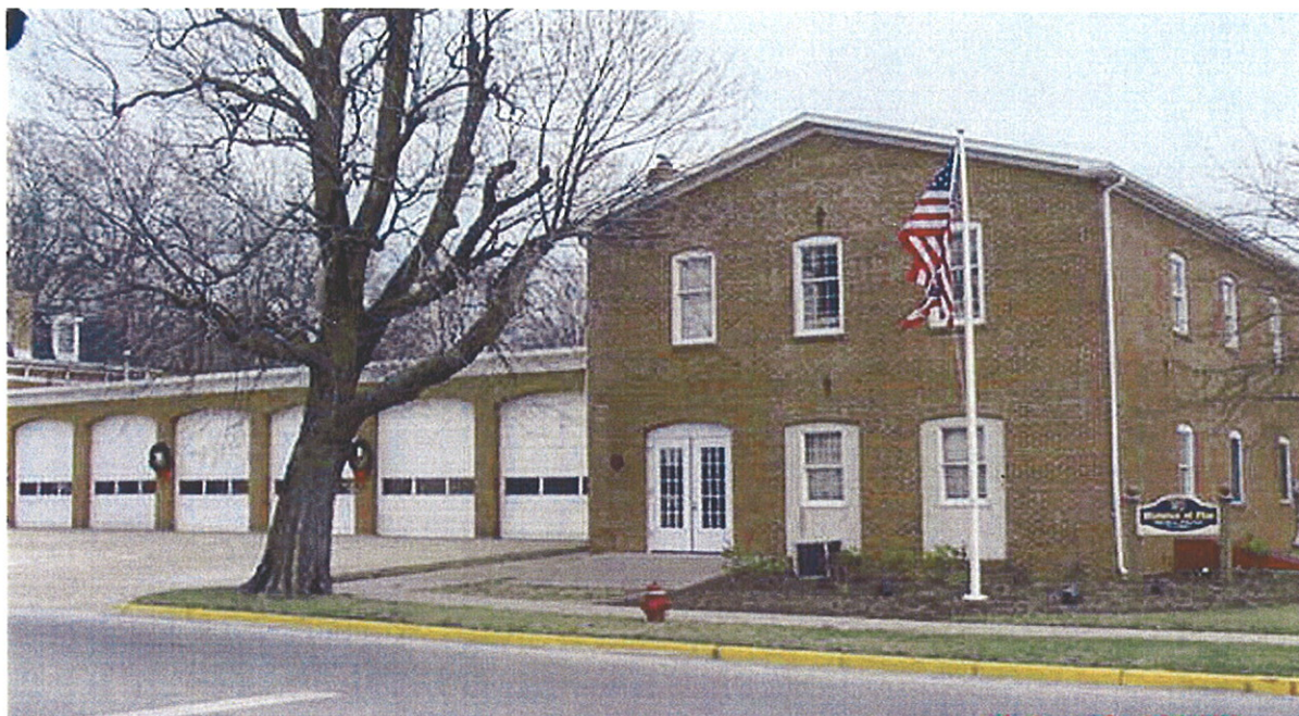
Photo #3: Oxford Fire Station, Front View
