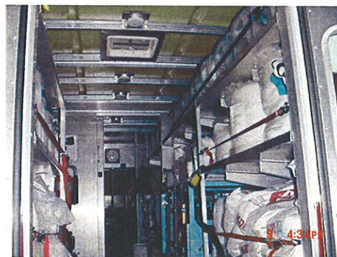
Photo #15: Task Unit Interior
